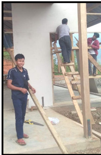
Installing the wall boards
