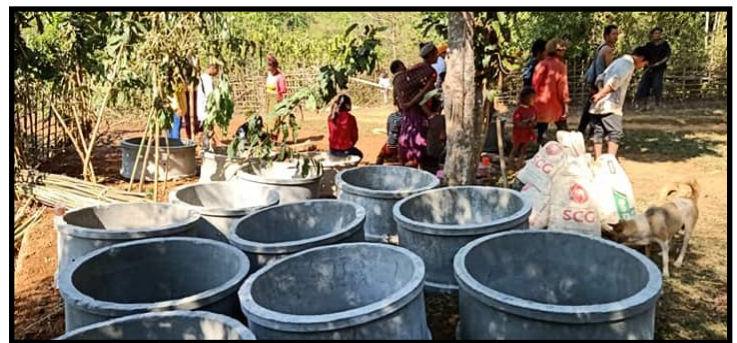
Preparing to make the well
