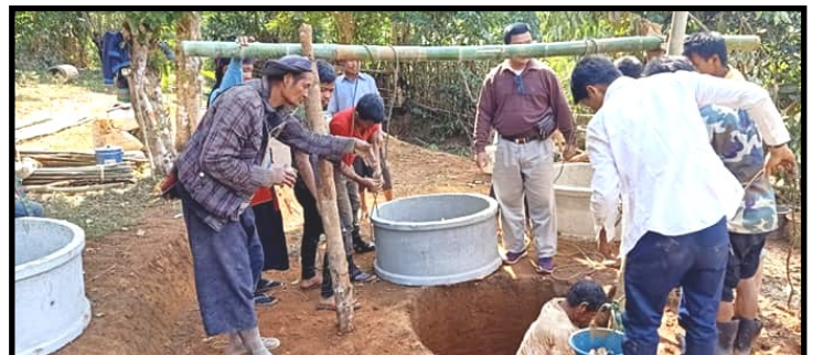
Lowering the well casing
