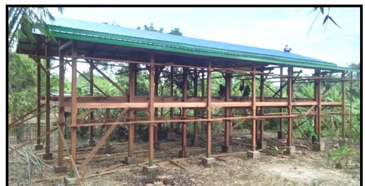
Finishing the Roof
