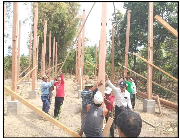
Raising the Timber Structure
