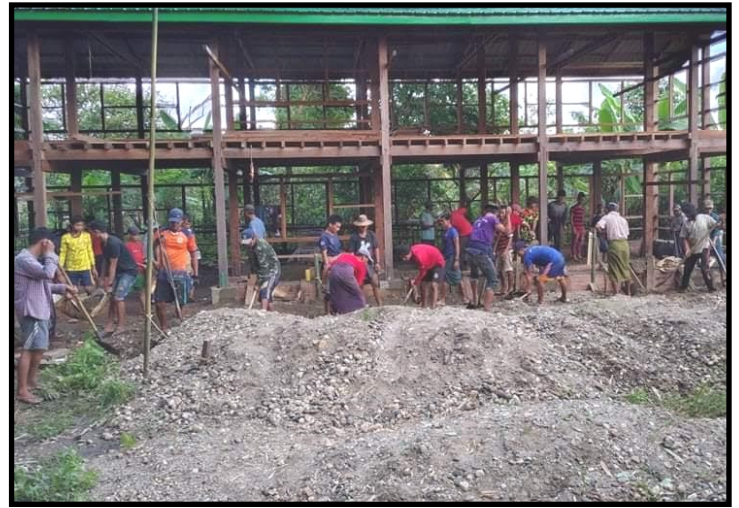
Working to Make the concrete Floor
