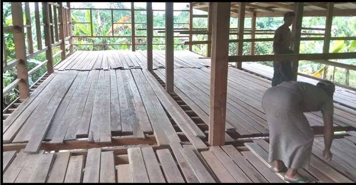
Drying The Floor Boards
